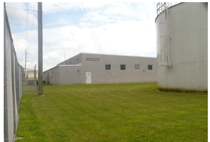
Borough of Kutztown Water Treatment Plant
