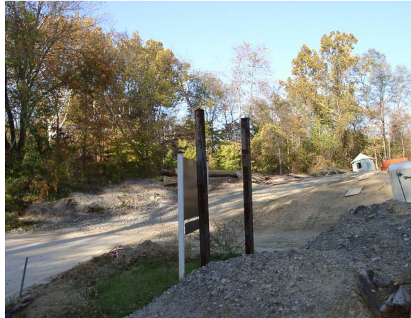
Figure VI-19 Old railroad grade removed for new development
