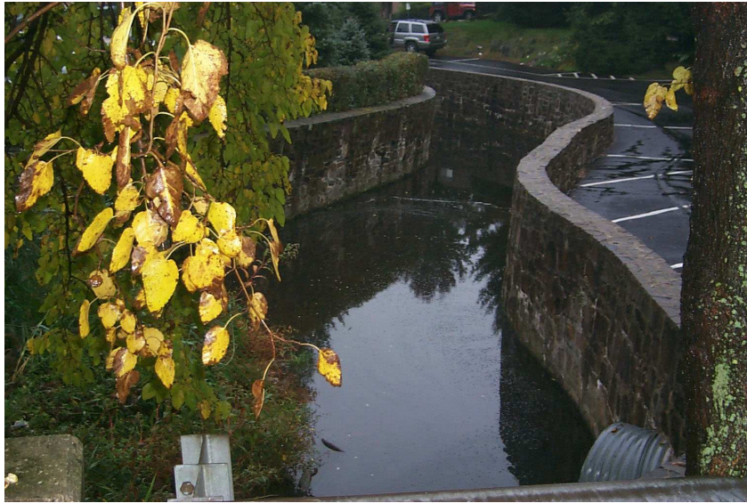
Figure IV-4 The Little Darby Creek off Sugartown Road in Radnor Township
