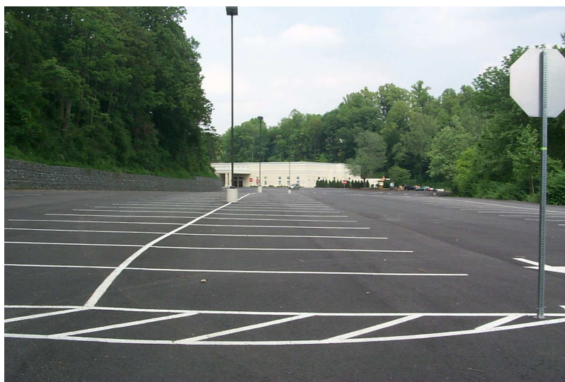
Figure IV-7 Floodplain Encroachment near Drexelbrook, main stem Darby Creek
