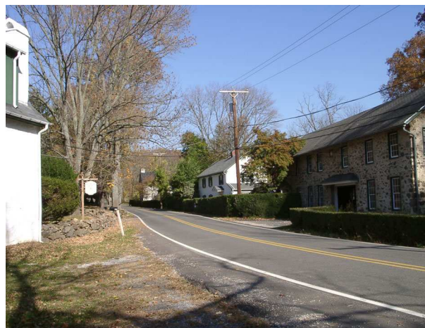
Figure VI-11 Waterloo Mills Historic District
