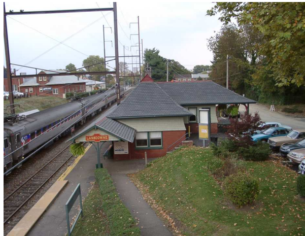
Figure VI-31 Historic Lansdowne Station
