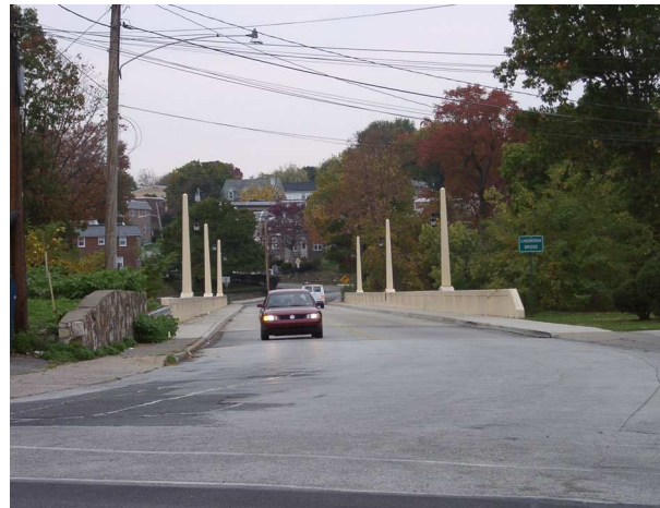
Figure VI-29 Restored Lindbergh Bridge
