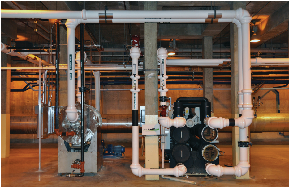
The Department's Sewage Geothermal Installation, located at the Southeast Water Pollution Control Plant.
