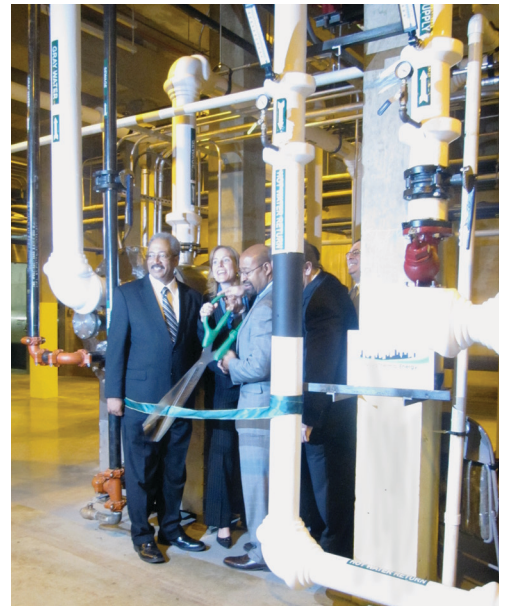
Mayor Michael A. Nutter cut the ribbon on the Sewage Geothermal Installation on April 12, 2012.
