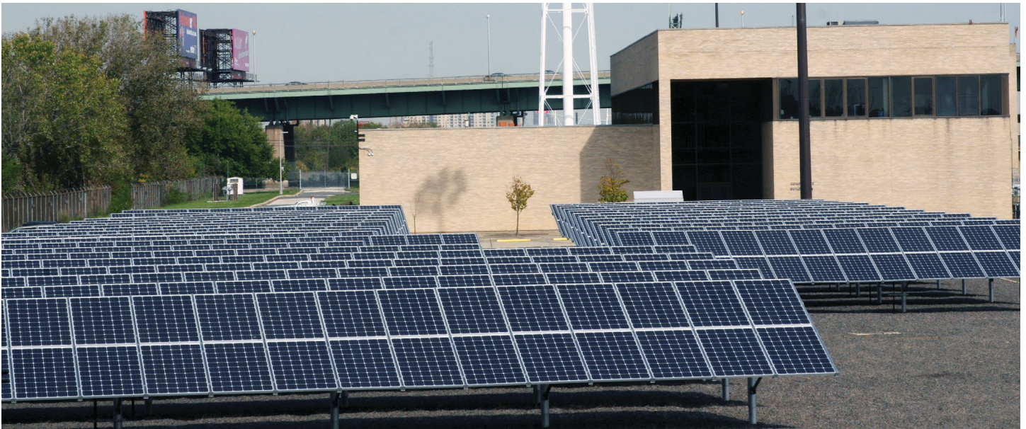
The Department commenced with the installation of its first solar panel system in August 2010. This system consists of 1,014 photovoltaic solar panels and is located at the Southeast Water Pollution Control Plant.
