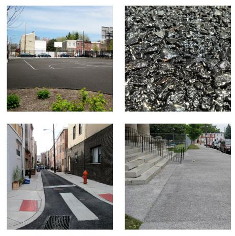
Figure 1-24. Examples of Pervious Paving in Philadelphia
