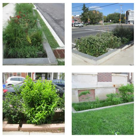
Figure 1-5. Examples of Stormwater Planters in Philadelphia
