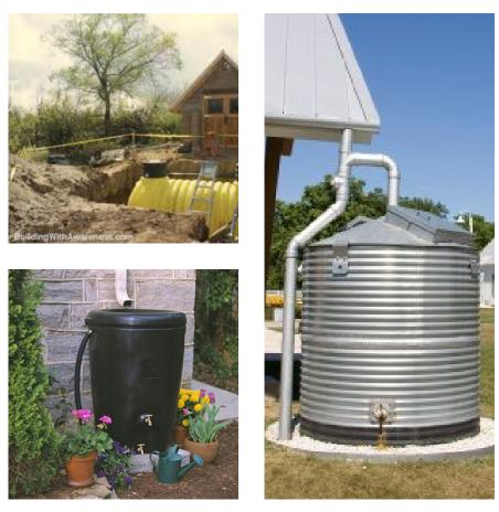
Figure 1-20. Examples of Cisterns and a Rain Barrel
