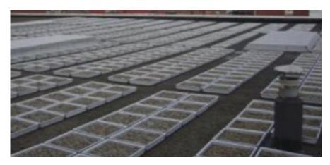
Figure 1-26. Examples of Blue Roofs in New York City (Image credit: 2012 NYC Green Infrastructure Pilot Monitoring Report)
