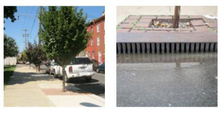
Figure 1-18. Examples of Stormwater Trees in Philadelphia
