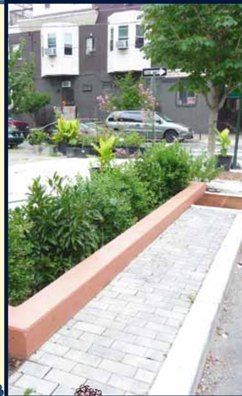
An example of a sidewalk stormwater planter located in Philadelphia
