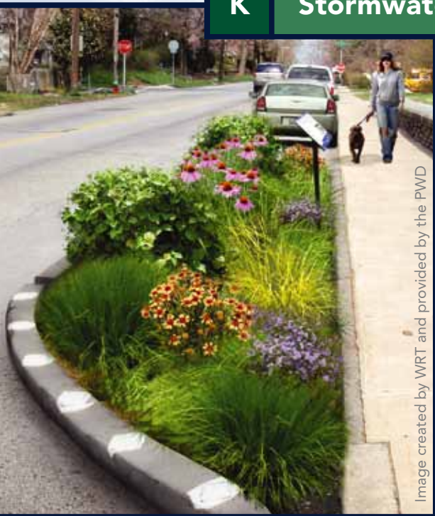
Example of a stormwater curb bumpout in Philadelphia
