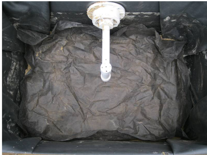
3. Filter fabric installed overtop gravel.
