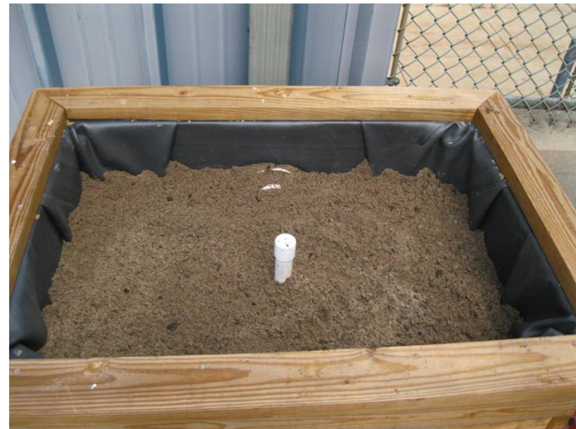
4. Soil mix (12 inches) installed with space for overflow stick up.
