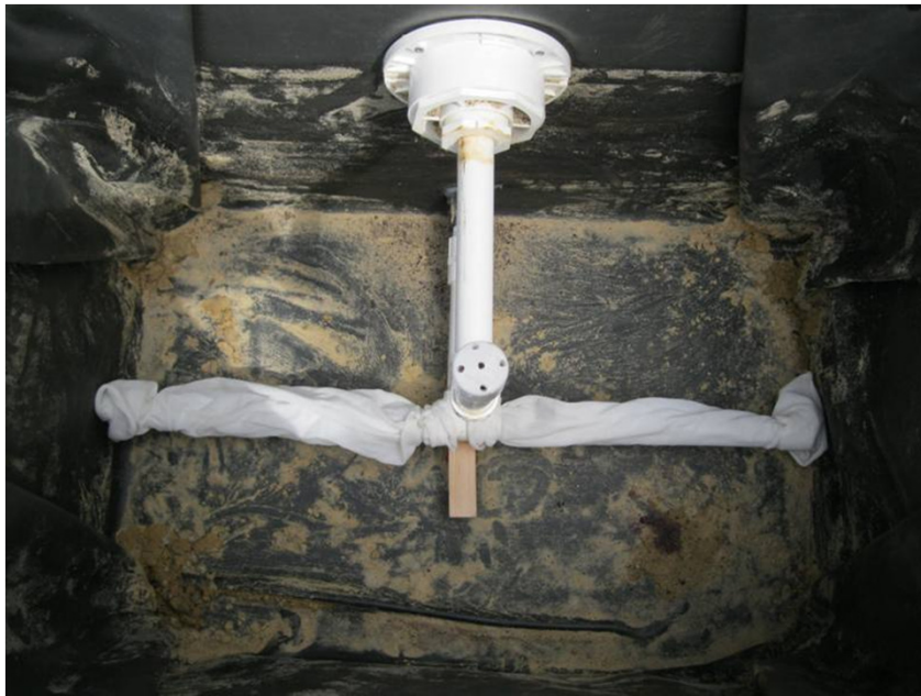
1. Underdrain (w/fabric) & overflow plumbing installed.
