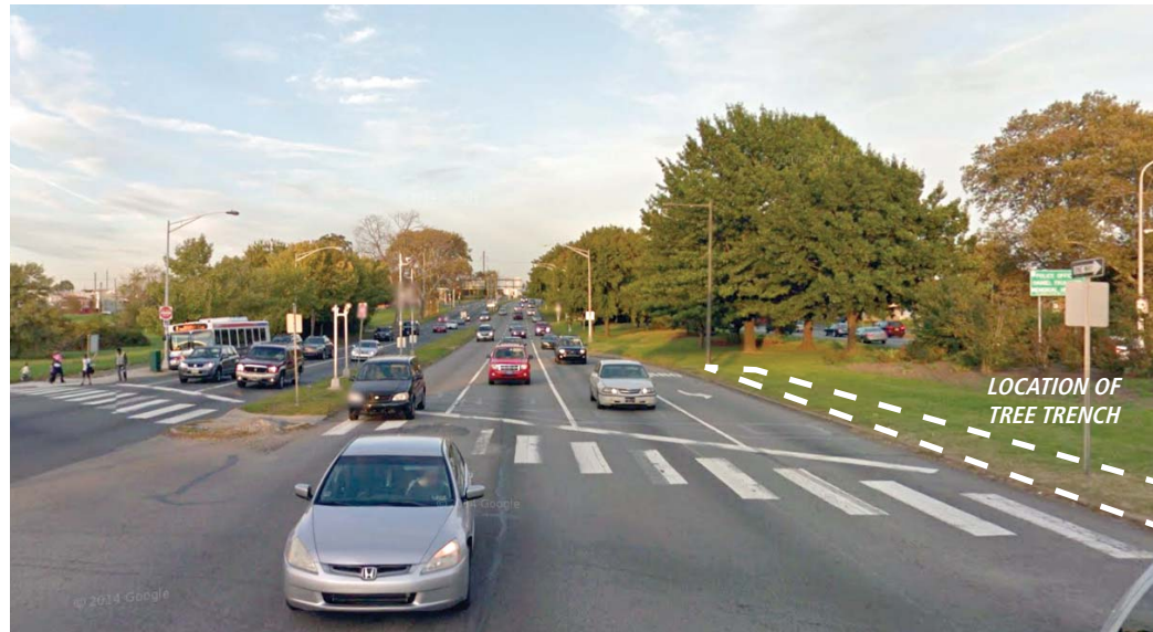
Boulevard - Existing Conditions
