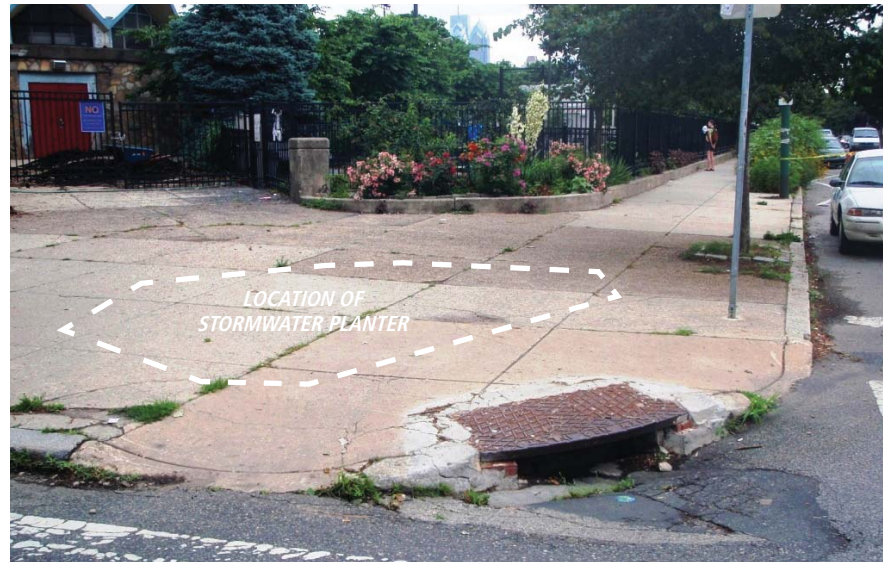
Park Sidewalk - Pre-construction Conditions
