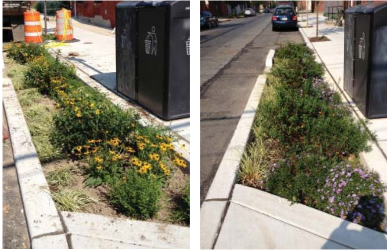
Figure 3-5. Example of a Stormwater Bump-out in Summer and Fall. Bump-out includes flowers that bloom at different times to create interest in different seasons.
