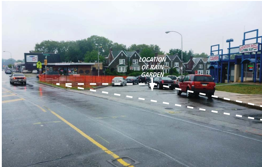
Traffic Triangle - Pre-construction Conditions
