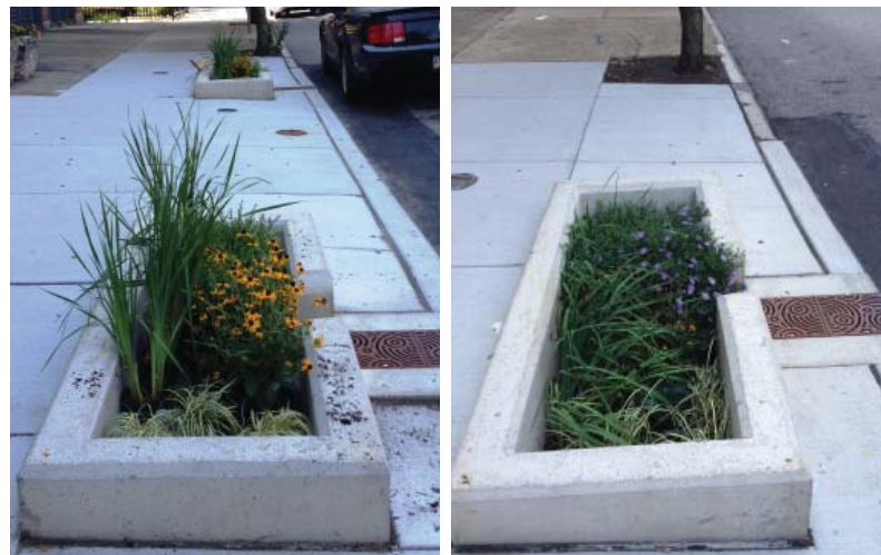
Figure 3-4. Example of a Stormwater Planter in Summer and Fall. Planter includes flowers that bloom at different times to create interest in different seasons.
