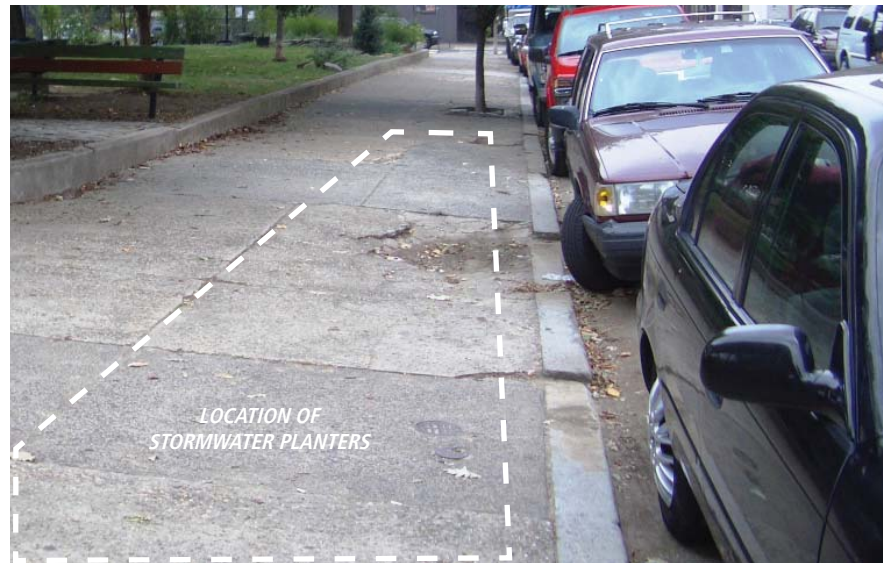
Stormwater Planter - Pre-Construction Conditions
