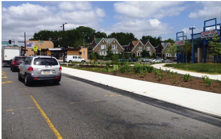
Traffic Triangle - Post-construction Conditions
