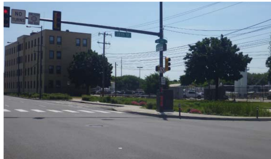
Industrial Street - Post-Construction Conditions
