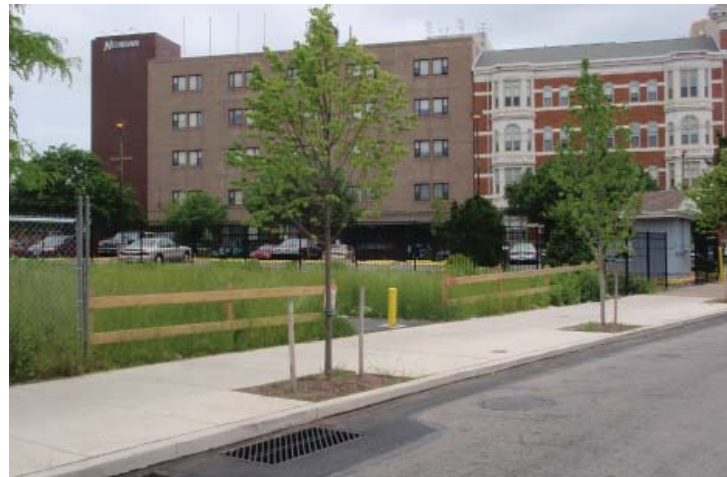
Figure 3-1. Examples of Stormwater Tree Trenches in Philadelphia
