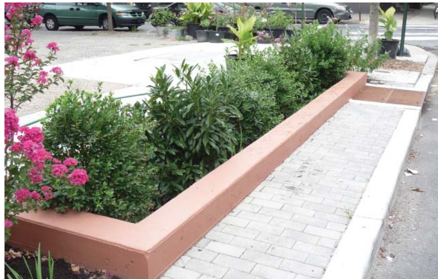
Stormwater Planter - Post-Construction Conditions
