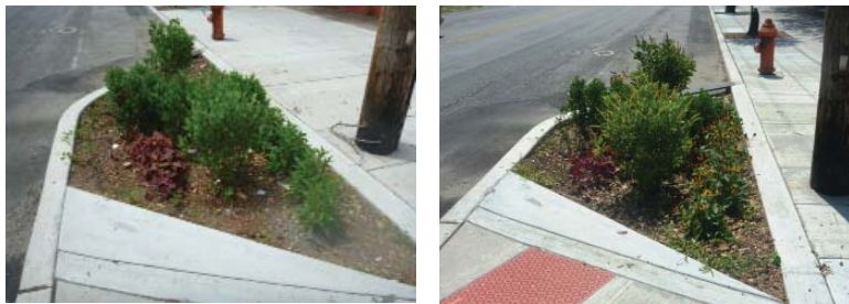
Figure 3-6. Example of a Stormwater Bump-out in early Spring and late Summer. Shrubs provide structure while blooms accent the planting.
