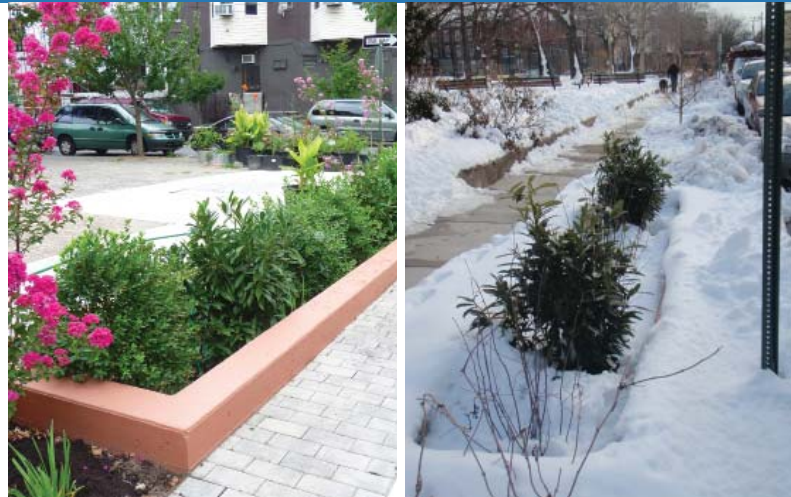
Figure 3-3. Example of a Stormwater Planter in Summer and Winter. Evergreen shrubs help to make the planter visible year-round.
