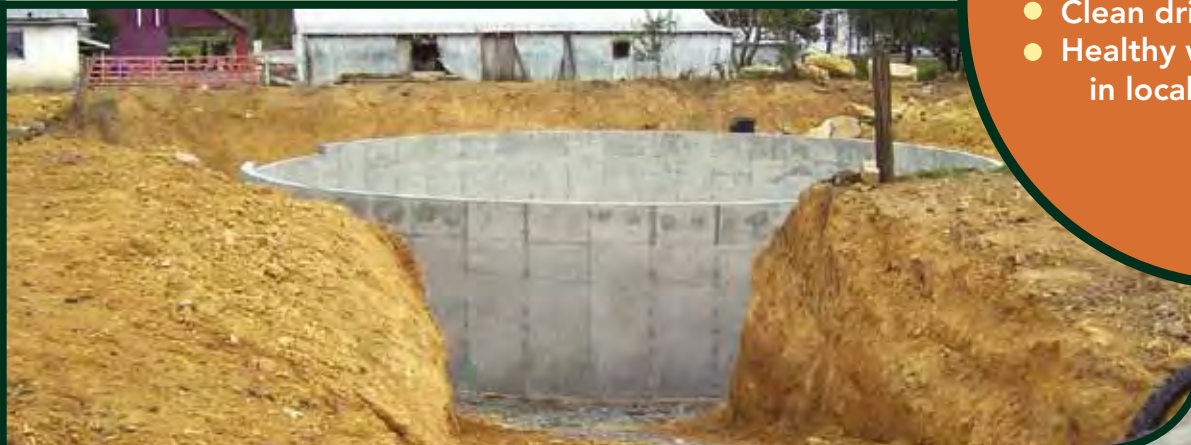
An in-ground liquid manure tank during construction.
