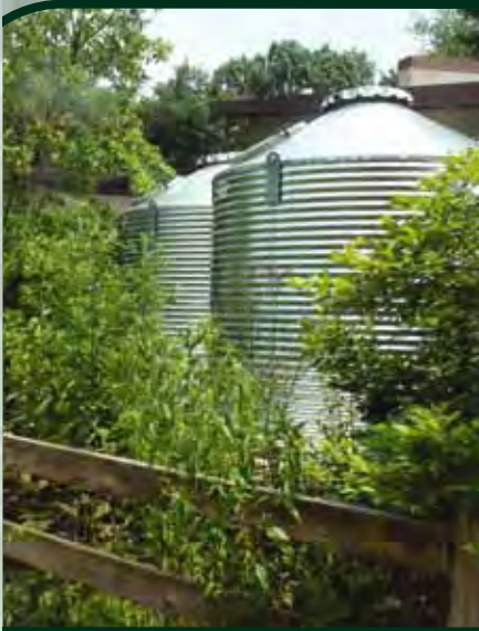
Two cisterns at the Schuylkill Center for Environmental Education in Philadelphia, PA capture runoff from the education building roof.
