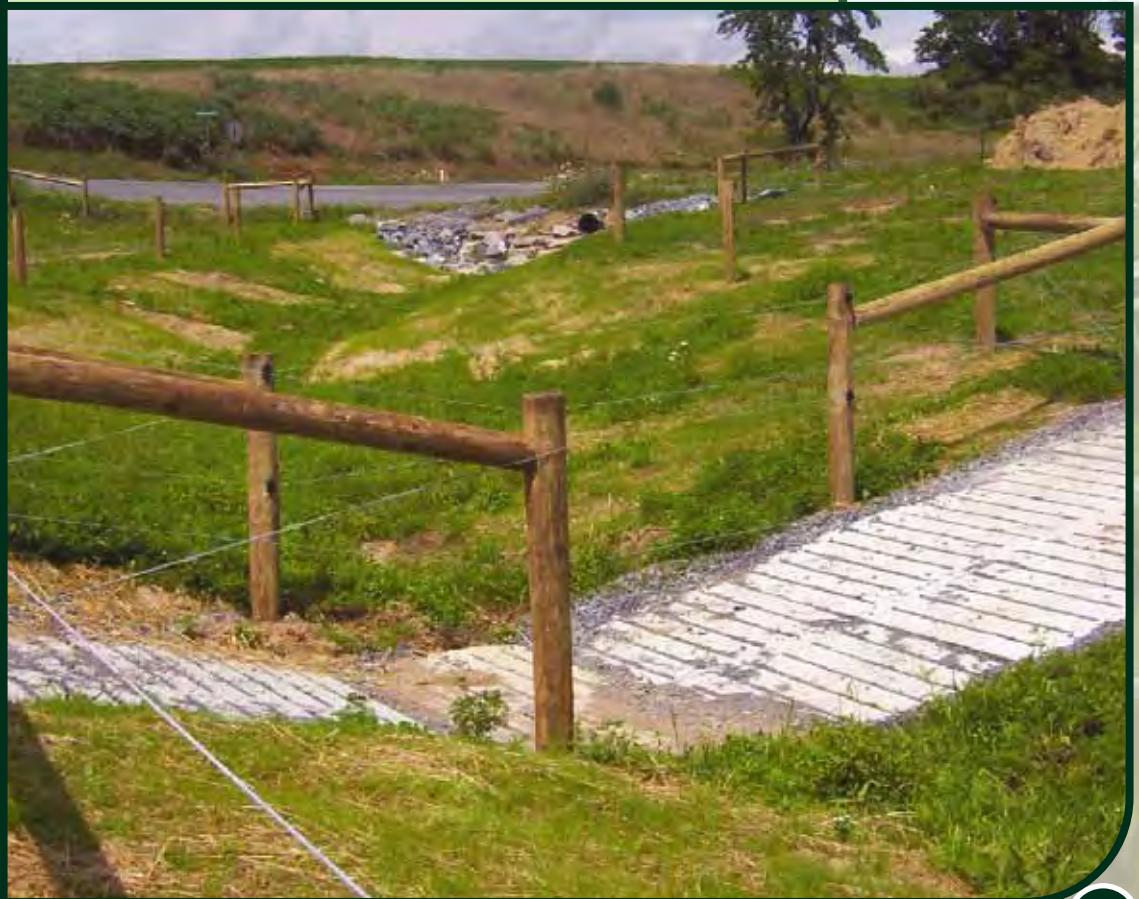
Cattle crossings help reduce soil loss, protect water quality and prevent cattle and equipment from getting stuck.
