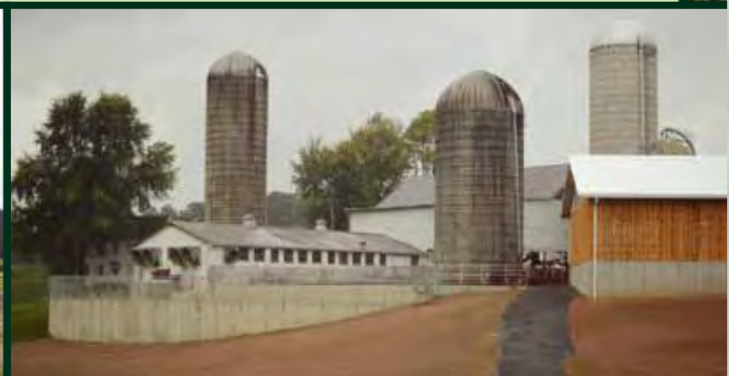
This farm has a liquid manure storage tank on the left and a dry manure storage facility on the right.
