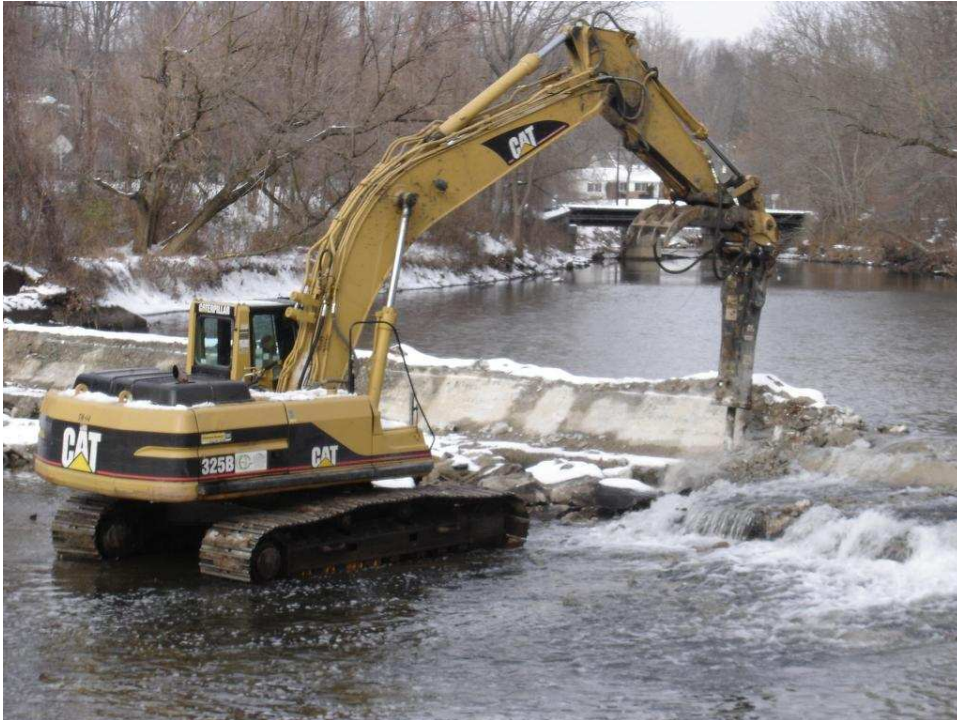
Figure O.1 Excavator in Process of Removing Bethayres Dam
