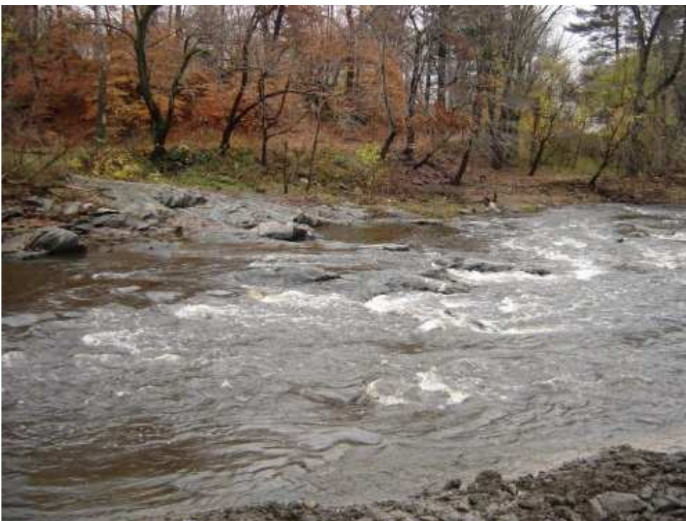
Figure O.4 Former Site of Frankford Avenue Dam after Removal Process
