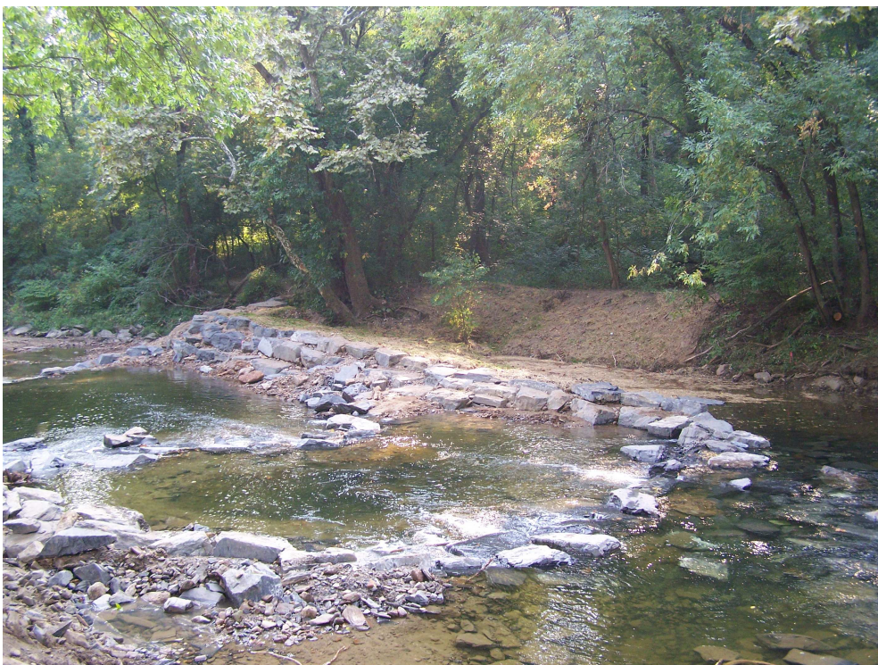
Figure O.10 Completed Pennypack Creek Rock Ramp Fishway
