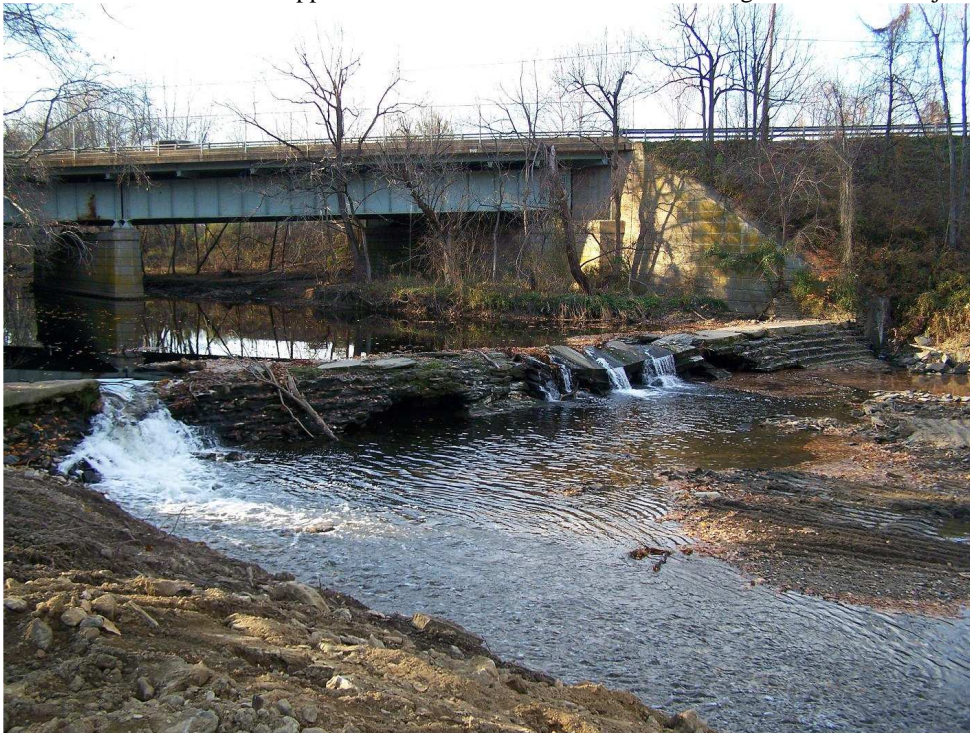
Figure O.5 Huntingdon Pike Dam Prior to Removal Process
