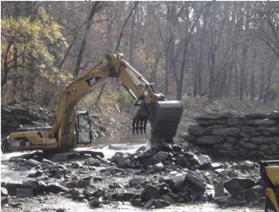
Figure O.7 PWD Contractor in Process of Removing Rhawn Street Dam
