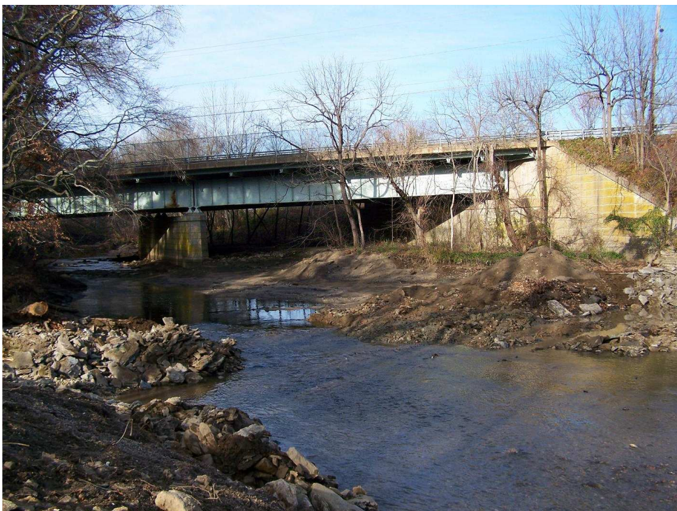
Figure O.6 Former Site of Huntingdon Pike Dam after Removal Process
