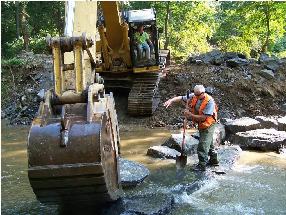
Figure O.9 Bill Weibrecht Arranging Boulders During Pennypack Creek Rock Ramp Construction
