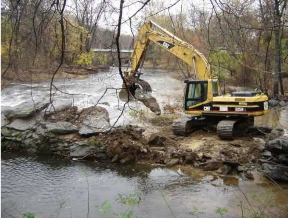
Figure O.3 PWD Contractor in Process of Removing Frankford Avenue Dam
