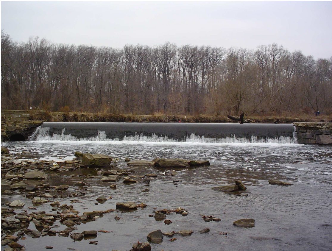
Figure N.2 Upstream View of Verree Road Dam
