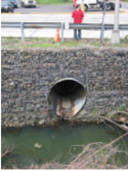
Wire Mesh Retaining Wall
