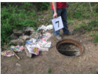
Missing Manhole Cover
