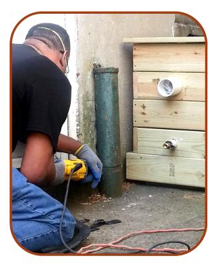
Using grinder and/or reciprocating saw, cut sewer riser to appropriate height, if necessary. From planter, all piping should maintain at least ¼" per every 4 feet of downward pitch for proper drainage. Exact height of riser cut will vary.
