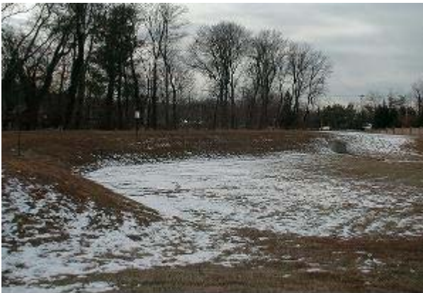
A dry extended detention pond is designed to temporarily detain runoff during storm events
