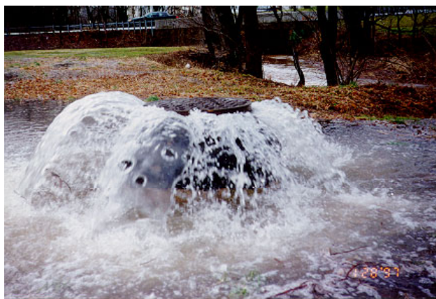
Figure 1.4.6-4 Overflowing Manhole Nearby a Stream
