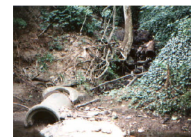
9. Dumped construction material along the banks, and invasive ivy prevent the riparian buffer from flourishing. Action/BMP : Determine who is routinely dumping to clean up, and replant the riparian buffer.
