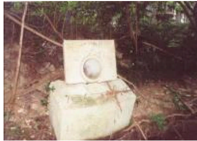
1. Dislodged/eroded drainage pipe behind Oak Summit Apartments (right bank) Action/BMP: Repair stormwater pipe
