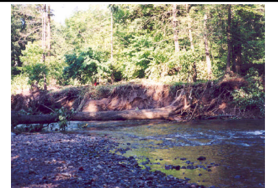
5. Newly eroded banks as a result of Tropical Storm Allison. Action/BMP : This area is undergoing biotechnical streambank restoration. Continue to monitor for knotweed re-infestation.
