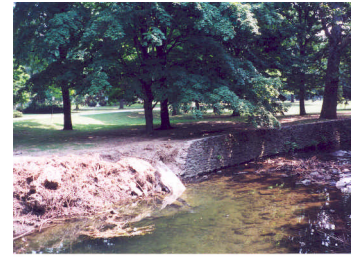
3. The stone walls constructed during the 1930's, are an attractive feature of the Tookany Creek Parkway. However, many areas have collapsed and are missing as the Tookany Creek has expanded its creek bed to accommodate the increasing volume of stormwater from the impervious surfaces in the upstream communities. Action/BMP : Conduct a complete study of the hydrology of the Tookany Creek using the Rosgen model to develop a long-term plan for the restoration.
