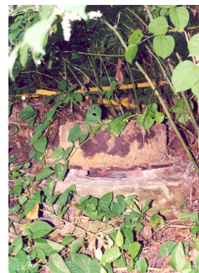
6. Broken/breached concrete collar of sanitary sewer Action/BMP: Have the township engineer assess the problem and develop solution
