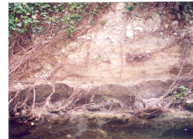
4. Vertical creek bank behind Oak Summit Apts., scouring of bank and undercutting Action/BMP: Develop a plan for biotechnical streambank restoration
