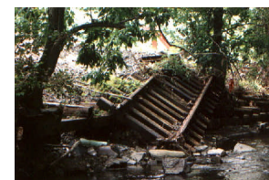
7. SEPTA leave its debris behind after track repairs. Action/BMP : Township will work with SEPTA to clean it up.
