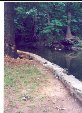
2. Typical mowed lawn up to the wall which prevents NPS pollution from being filtered by the riparian buffer and stabilizing the eroding channel bed Action/BMP : Replant the understory of shrubs and herbaceous layer along walled areas of the Tookany Creek.
