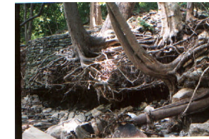
4. Tree roots are exposed along the steep banks behind the Wyncote Post Office due to severe runoff from surrounding parking lots of the train station and post office. Action/BMP : Consider an infiltration system at the end of the Jenkintown train station parking lot and post office.
