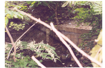
5. Broken concrete bulkhead Action/BMP: Have the township engineer assess the problem and develop solution.
