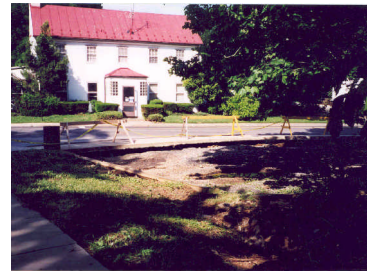
7. This intersection continually floods during storm events. This picture shows the severe damage to the road after Tropical Storm Allison in 2001. Action/BMP : Conduct a complete study of the hydrology of the Tookany Creek using the Rosgen model to develop a long-term plan for the restoration.
