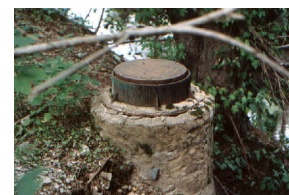
8. Exposed manhole from Tookany Creek bed down cutting and erosion. Action/BMP : Develop a program to inspect, repair and maintain manholes that are exposed.
