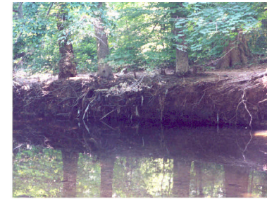
4. The steep wooded slopes of the west bank of the Tookany Creek along the Parkway are becoming undercut as a result of the upstream volumes of stormwater. The mature trees can hold the bank with their roots, but if the volume of water continues, the roots will be undermined and the trees will fall. Action/BMP : Conduct a complete study of the hydrology of the Tookany Creek using the Rosgen model to develop a long-term plan for the restoration. Use biotechnical streambank restoration to fortify the roots and stabilize the banks.
