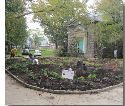
Volunteers plant the rain garden.
