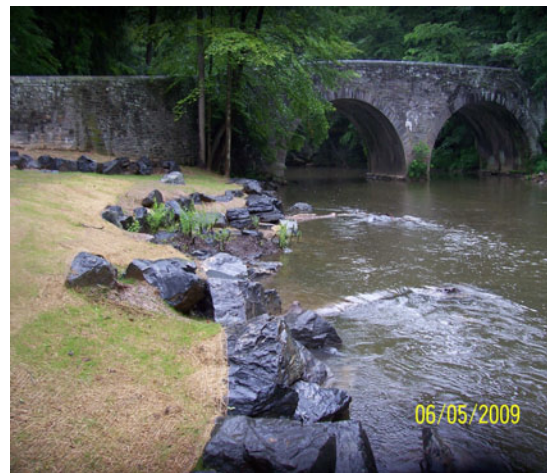
Figure 3-105: DSR bank in reach WSMS110 following emergency repairs (left); DSR bank following bank stabilization and instream flow structure installation (right).
