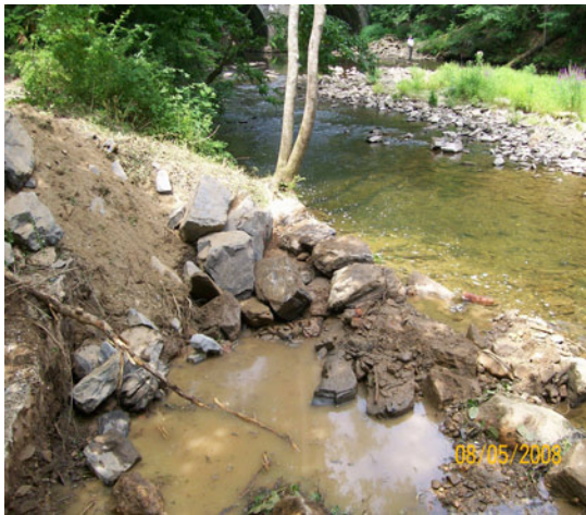
Figure 3-105: DSR bank in reach WSMS110 following emergency repairs (left); DSR bank following bank stabilization and instream flow structure installation (right).
