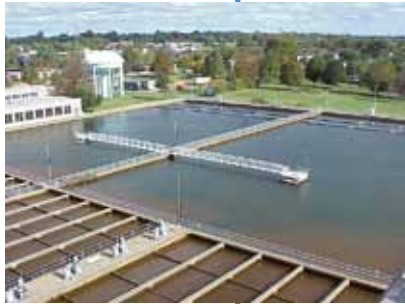
Baxter Water Treatment Plant
