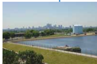
Queen Lane Water Treatment Plant
