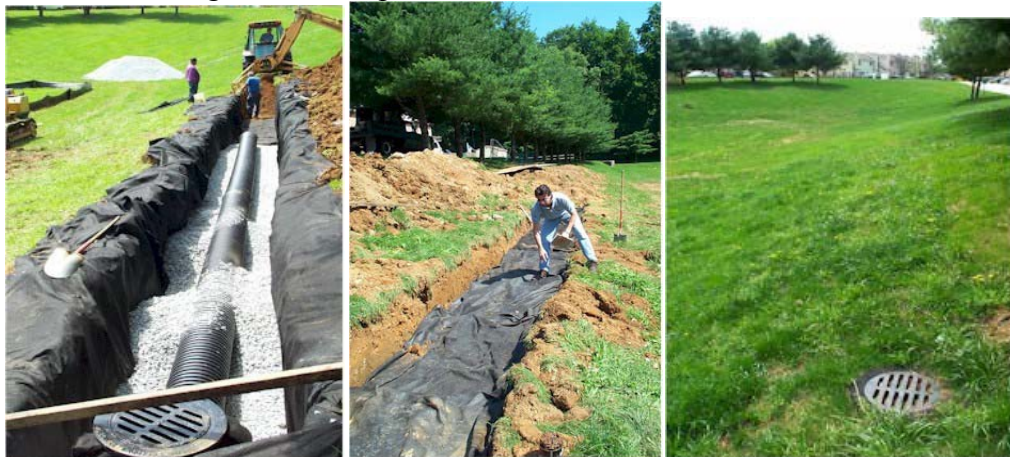
Figure 3: Example of Infiltration Trench Installation
