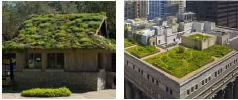
**Green Roof**: A vegetated surface installed over an existing roof surface. Vegetated roofs are effective in reducing the volume and velocity of stormwater runoff. A typical green roof consists of a waterproofing and root barrier layer, insulation, drainage and filter layer, growth media, and plants. Green Roofs can either be installed as a fixed structure or as a series of removable modules.
