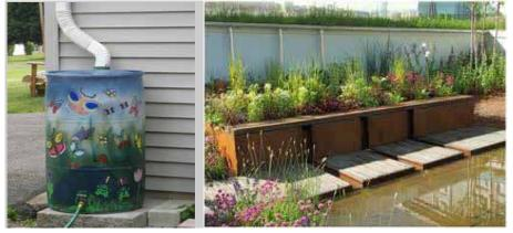
**Rain Barrel/Cistern**: A storage device that captures and stores runoff from roof leaders and is effective in reducing runoff volume from small storms. Stored water may be discharged to a pervious area, or treated and distributed to serve a variety of on-site water needs (ex: irrigation). Functions to the design potential when device is properly emptied after storm events.
