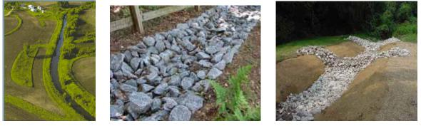
**Swale**: A vegetated basin designed to convey, attenuate and/or infiltrate stormwater runoff. In some cases, they are used to enhance water quality benefits. Porous media can be added to the swale base to enhance infiltration and water quality benefits.
