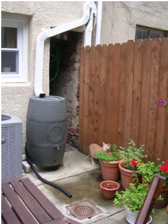
A rain barrel installed in the backyard of a South Philadelphia home.
