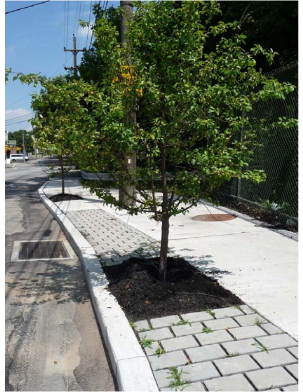
Stormwater Tree Trench
