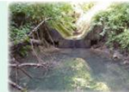
Bells Mill Stream Restoration Wissahickon Creek Watershed
