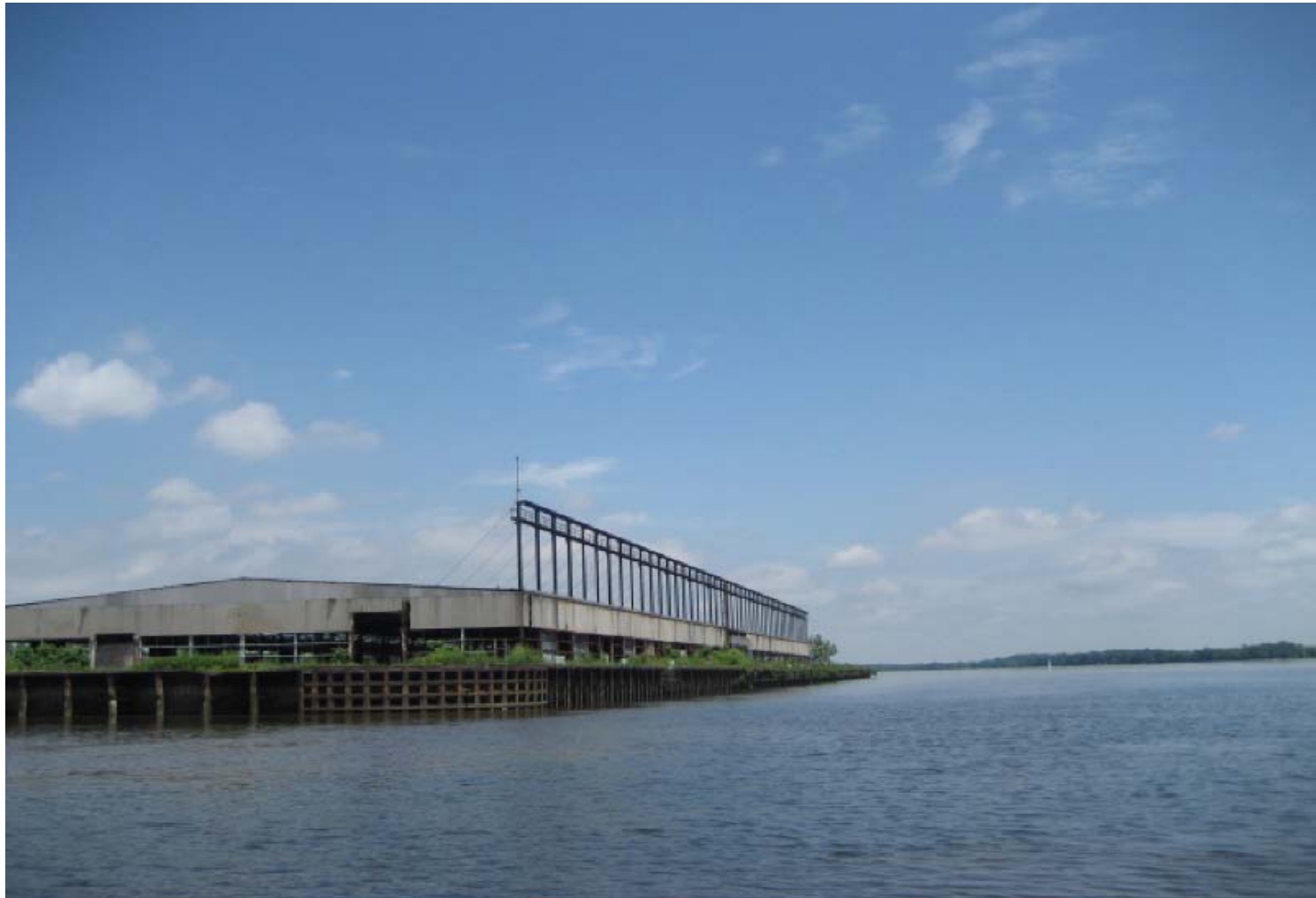
Abandoned Commercial/Industrial Site
