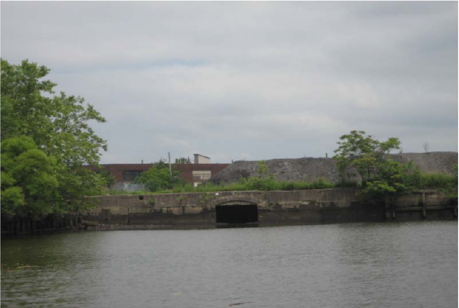
Storm Sewer Outfall
