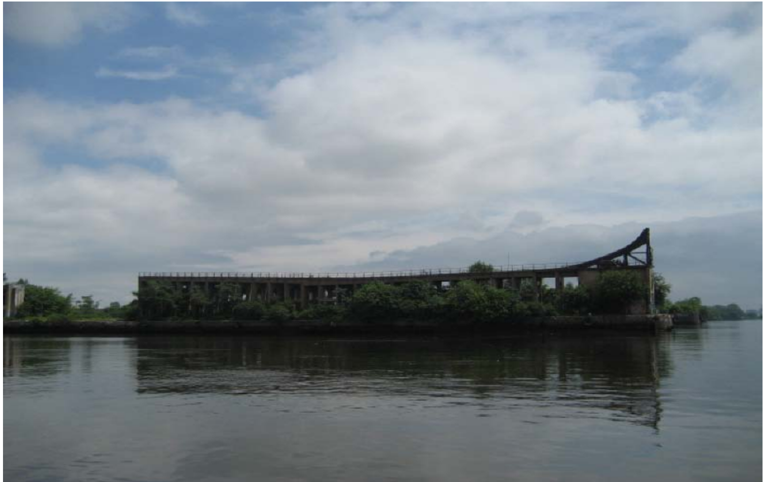
Abandoned Coal Receiving Dock
