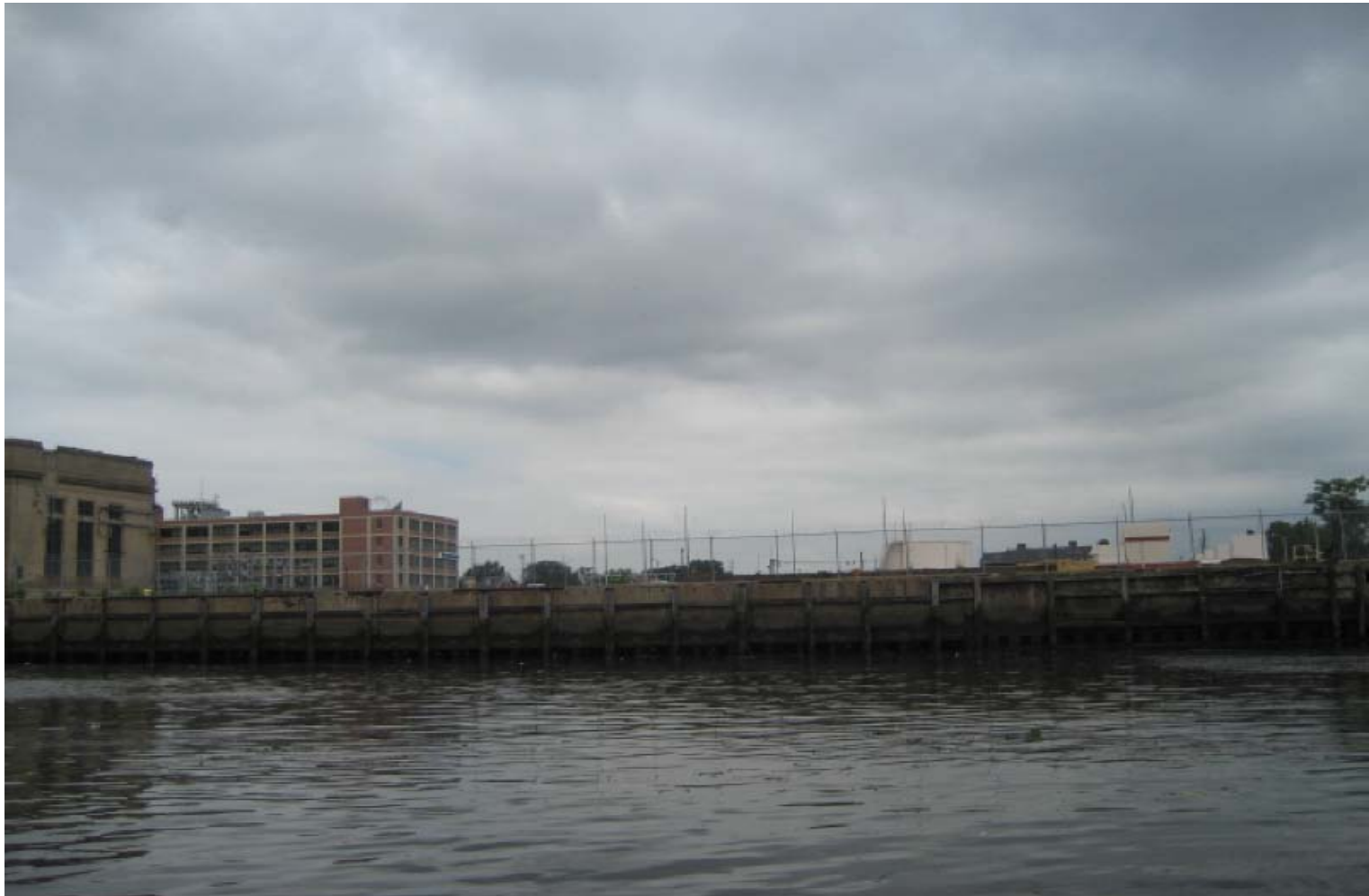
Bulkheaded Parking Lot
