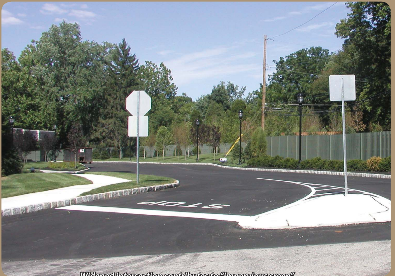
Widened intersection contributes to “impervious creep”
