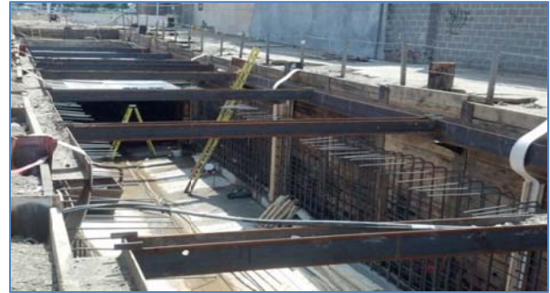
Typical Box Sewer Construction
